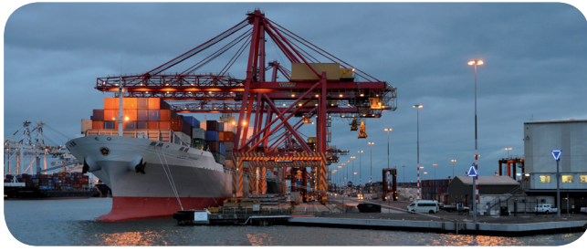
Swanson Dock, Port of Melbourne, Australia
